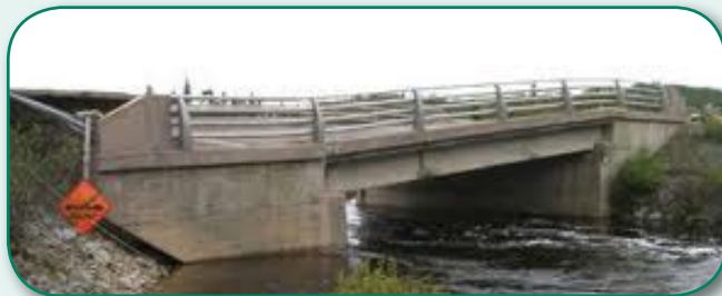
Rattle Brook Bridge - Damaged by Hurricane Igor
